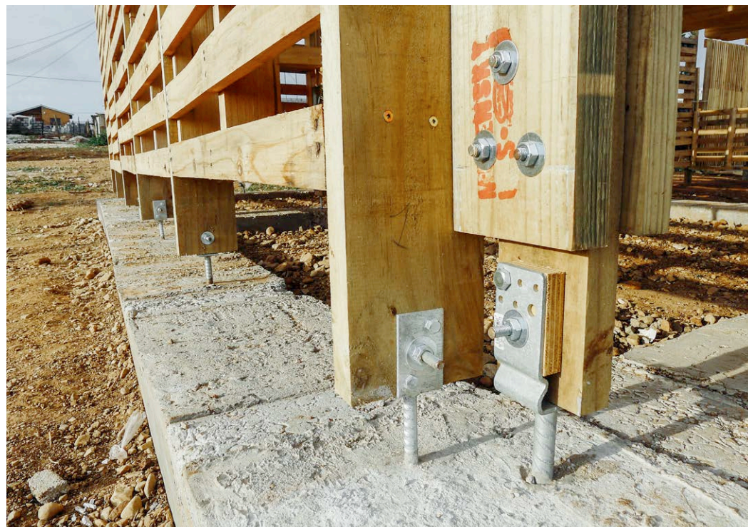
Base Fittings and Bolting Connections
