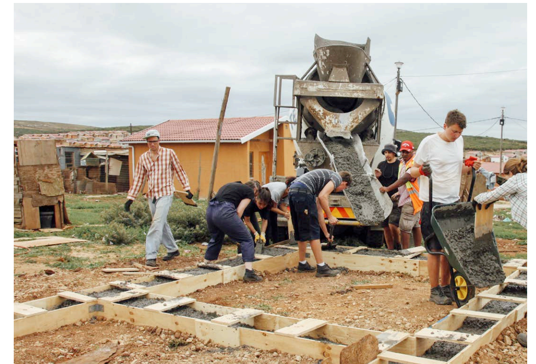
Pouring of Concrete
