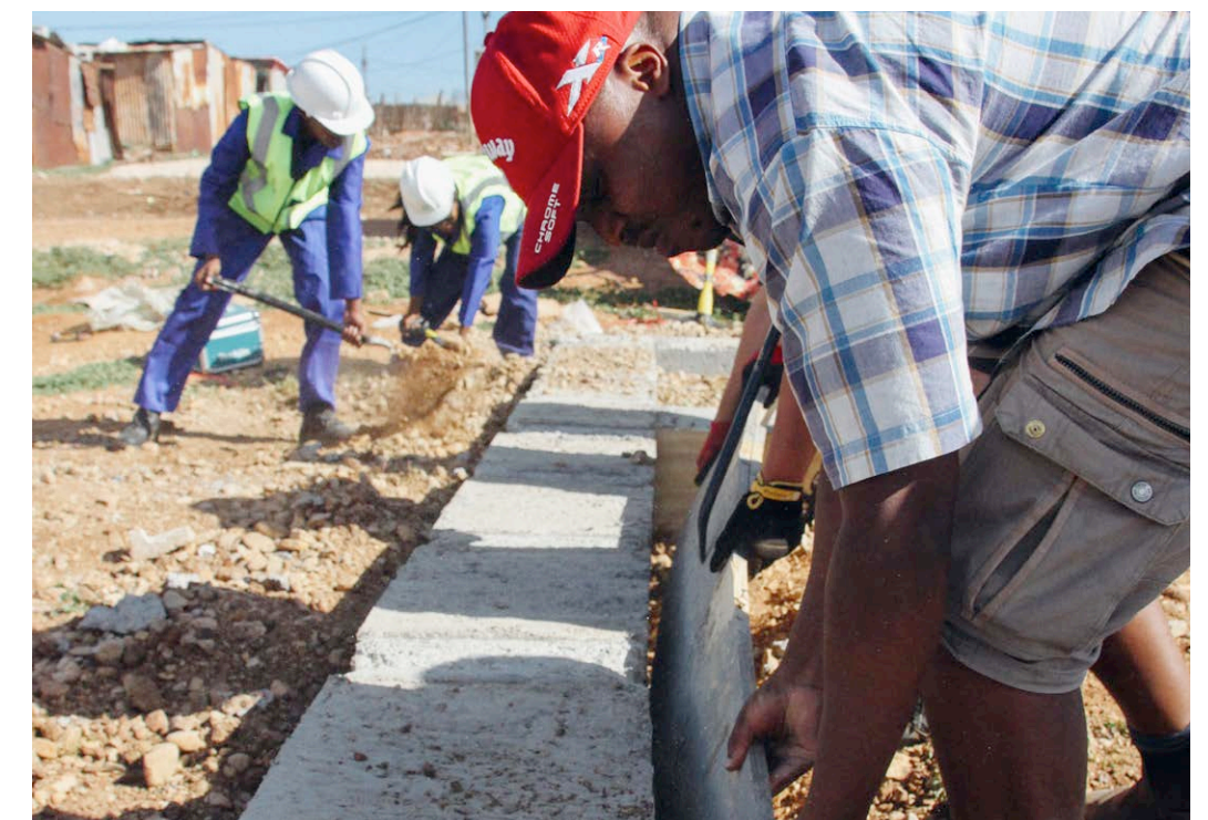
Stripping of Formwork and Backfilling
