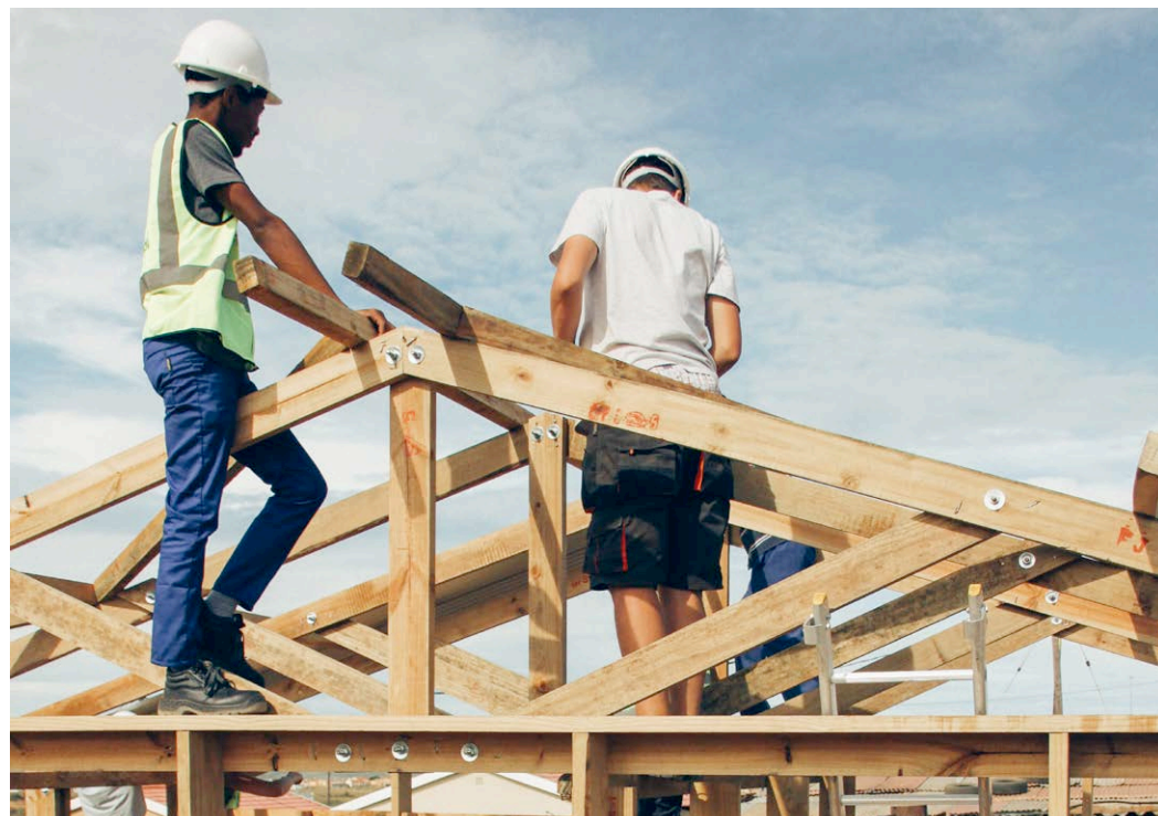
Placement of Purlins and Bracings
