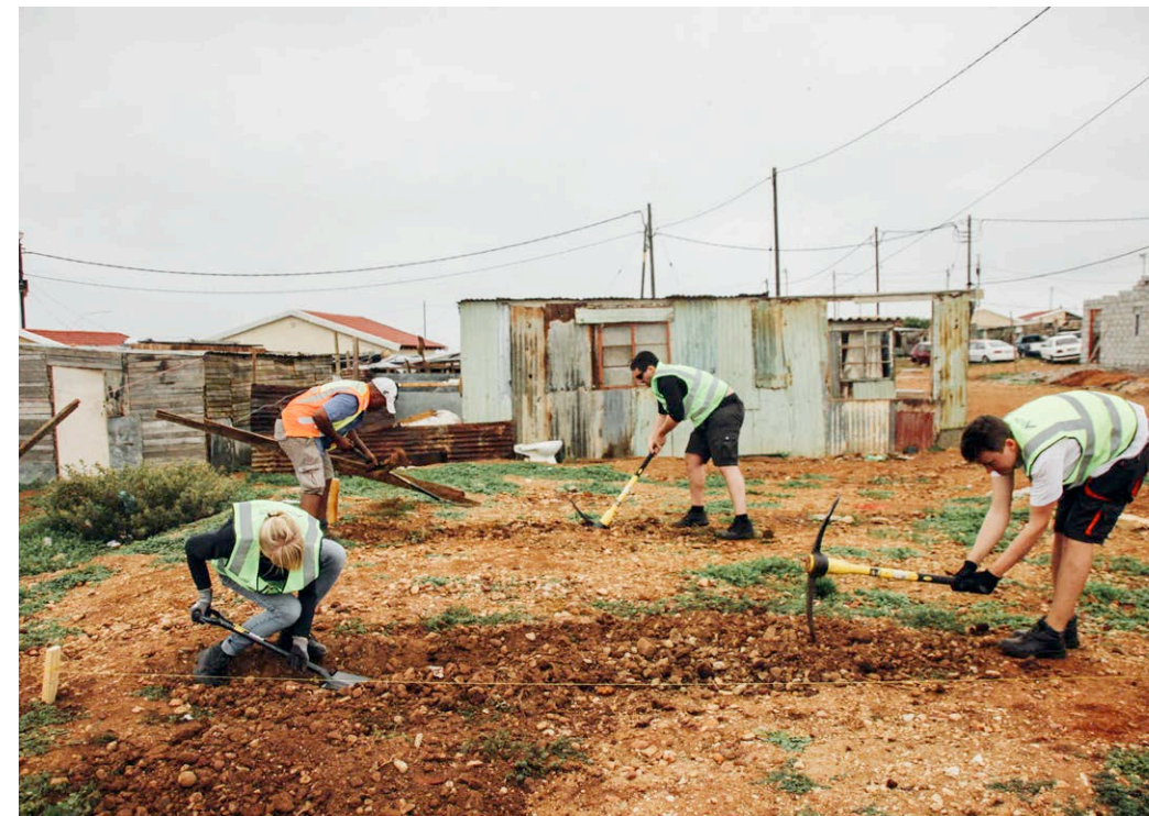
Setting up of Trenches for Strip Foundation
