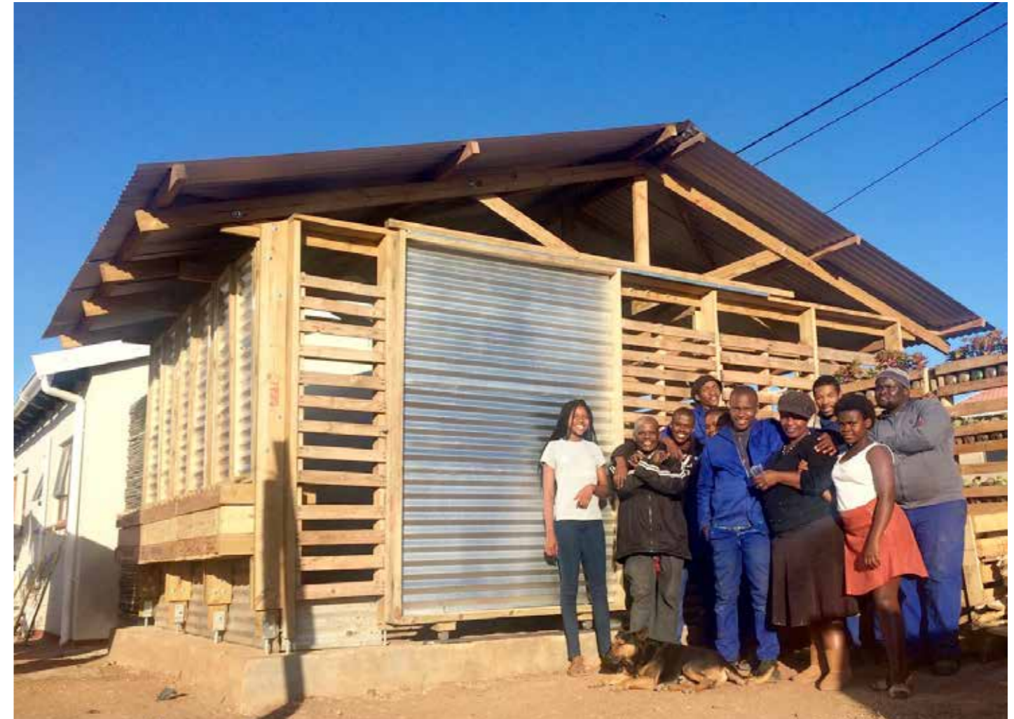
Hilda with PE College students after installation of a sliding door photo: Kevin M Kimwelle, May 2017
